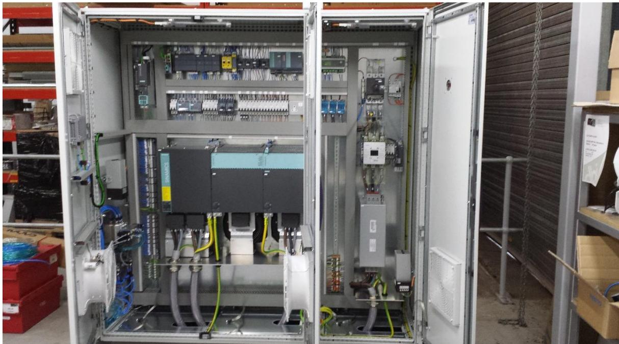
Figure 4 The Control Cabinet including Variable Speed Drive and PLC control system
